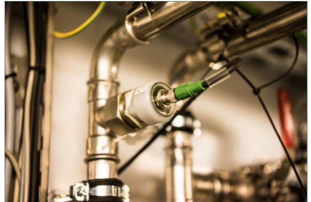
Conductivity measuring point with CONDIX4623
