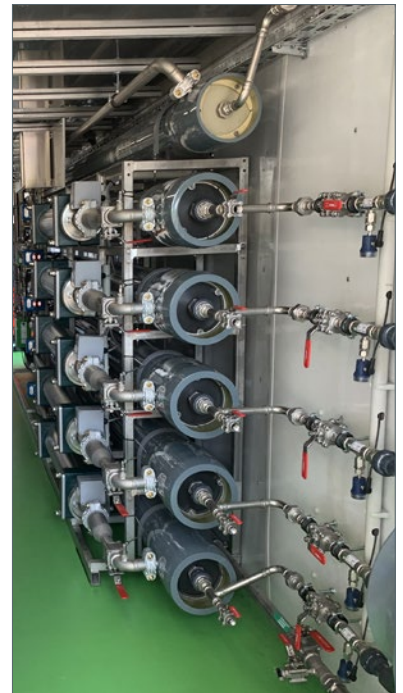
View into the container of the semi-permeable membranes of the RO system
